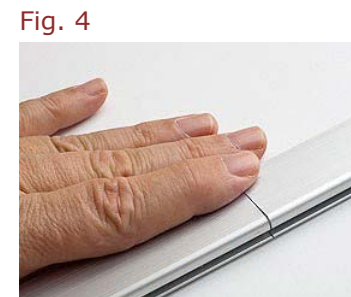
Fig. 3 Where tracks meet, the joint should be located at the centerline of the wall mount to ensure proper alignment.
